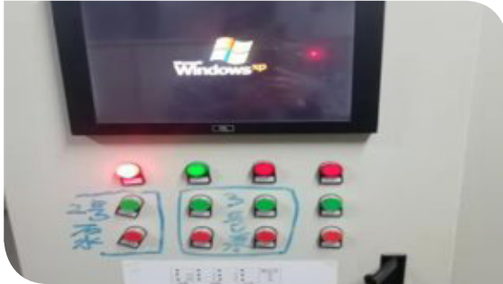
A frequency conversion system of the screw water pump in the central air-conditioning system is installed in Regal Jinfeng Hotel, which can save electricity consumption by 50% or above.
