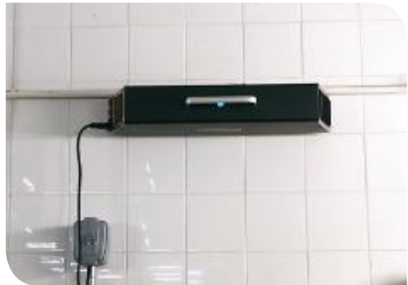
UV air sterilisation device for garbage room – We Go MALL
