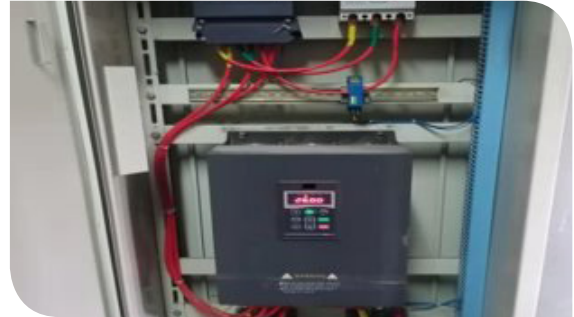
A frequency conversion system of the screw water pump in the central air-conditioning system is installed in Regal Jinfeng Hotel, which can save electricity consumption by 50% or above.
