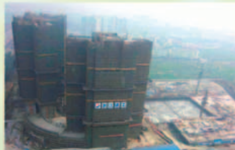
■ Structural frames of the three residential towers of first stage of the composite development have been completed
