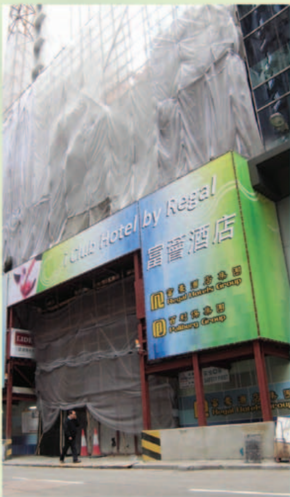
■ Superstructural works of the hotel development at 14 - 20 Merlin Street, North Point, Hong Kong in progress
