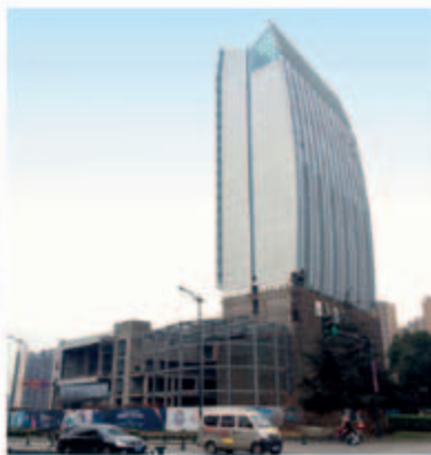
■ Regal Xindu Hotel, a five-star hotel in the first stage of the composite development - superstructure works in progress
