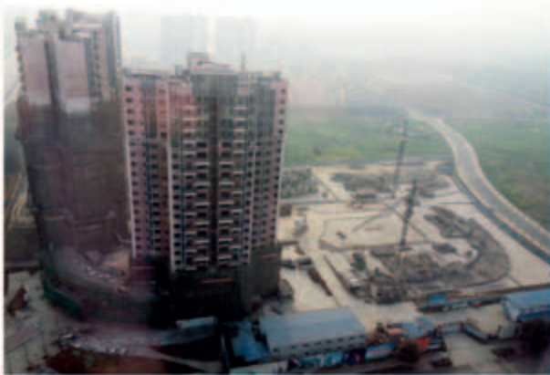
■ Three residential towers in the first stage of the composite development - superstructure works in progress
