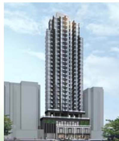
■ Commercial/residential development at Nos. 69-83 Shun Ning Road, Sham Shui Po, Kowloon – superstructure works in progress (*)
