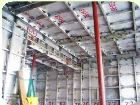
Aluminum formwork are used for the construction of typical floors to reduce timber use
