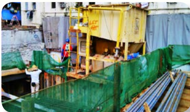
Wastewater treatment facilities at construction site
