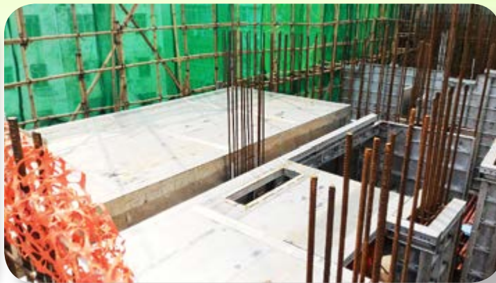
Aluminum formwork are used for the construction of typical floors to reduce timber use
