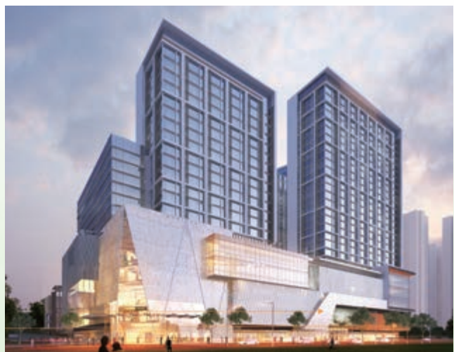
Commercial/office towers of Regal Cosmopolitan City (*)
