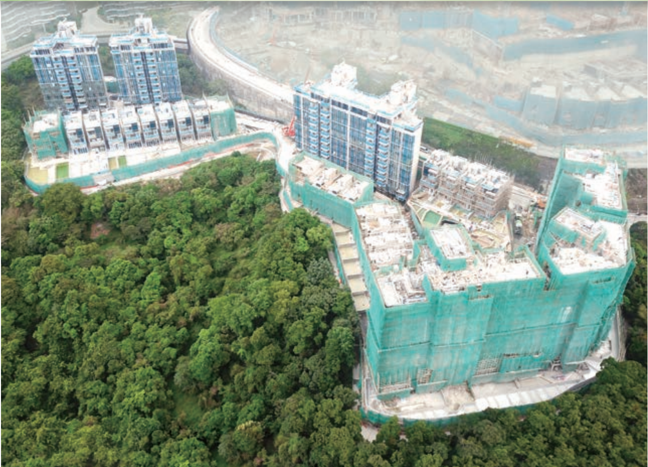
Luxurious residential development at Sha Tin Town Lot No. 578, Area 56A, Kau To, Sha Tin, New Territories – superstructure works in progress
