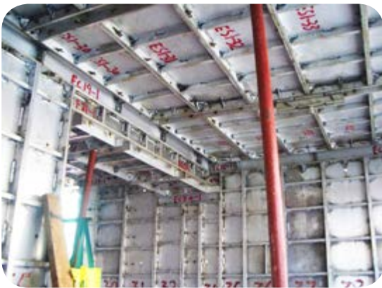
Aluminium formwork is used for the construction of typical floors to reduce timber use.
