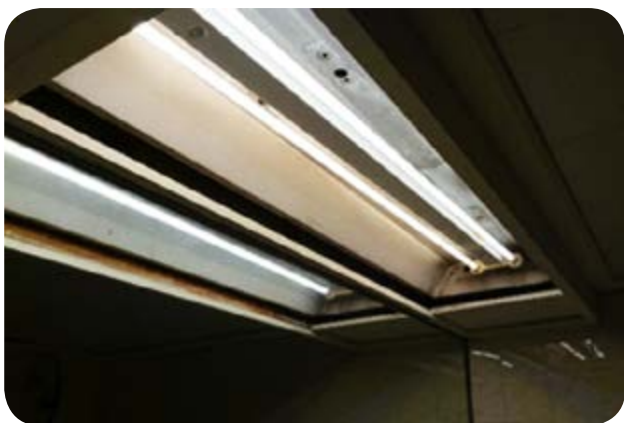
Regal replaced or are in the process of replacing the T8 fluorescent tubes in the guestrooms and public area with LED light tubes for further energy saving.
