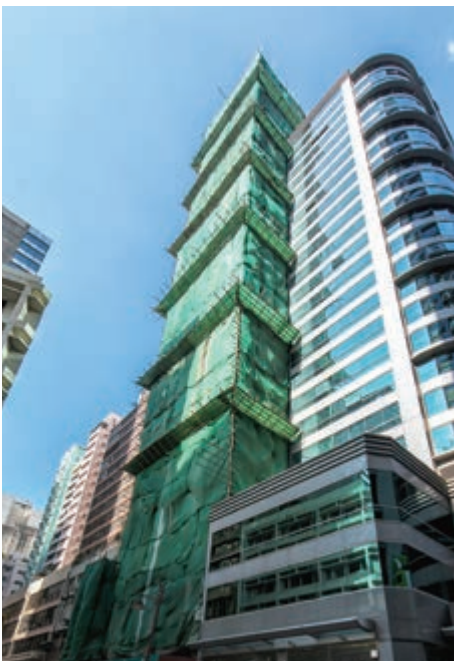
Nos. 5-7 Bonham Strand West and Nos. 169-171 Wing Lok Street, Sheung Wan intended to be named as "iclub Sheung Wan II Hotel" – superstructure works substantially finished
