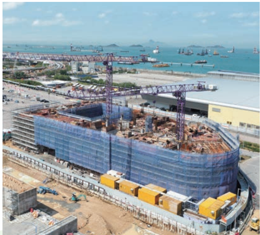
Regala Skycity Hotel – superstructure works in progress
