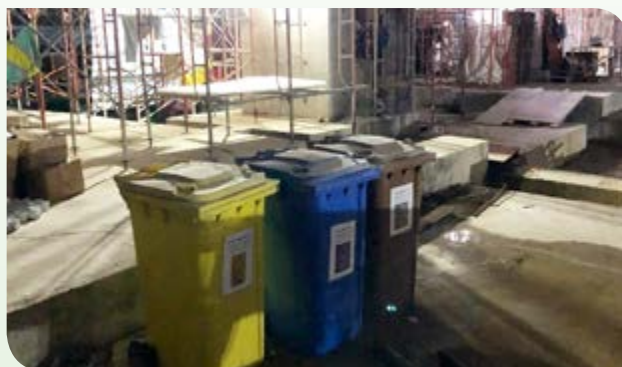
On-site waste sorting area
