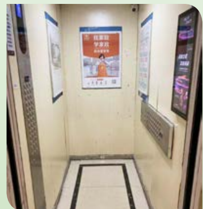
Tianjin Project added elevator button at appropriate height for the disabled.
