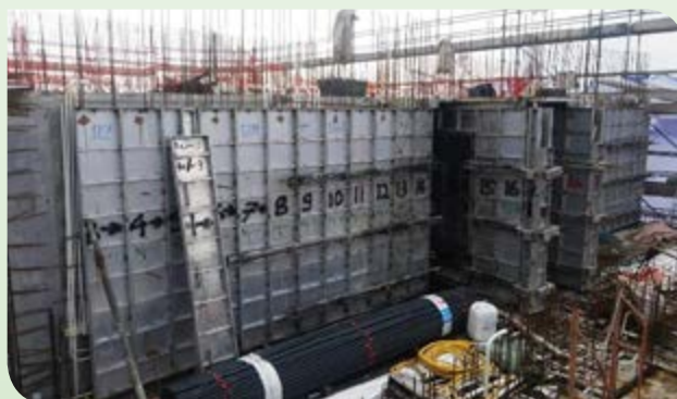
Aluminium formwork is used for the construction of typical floors to reduce timber use.
