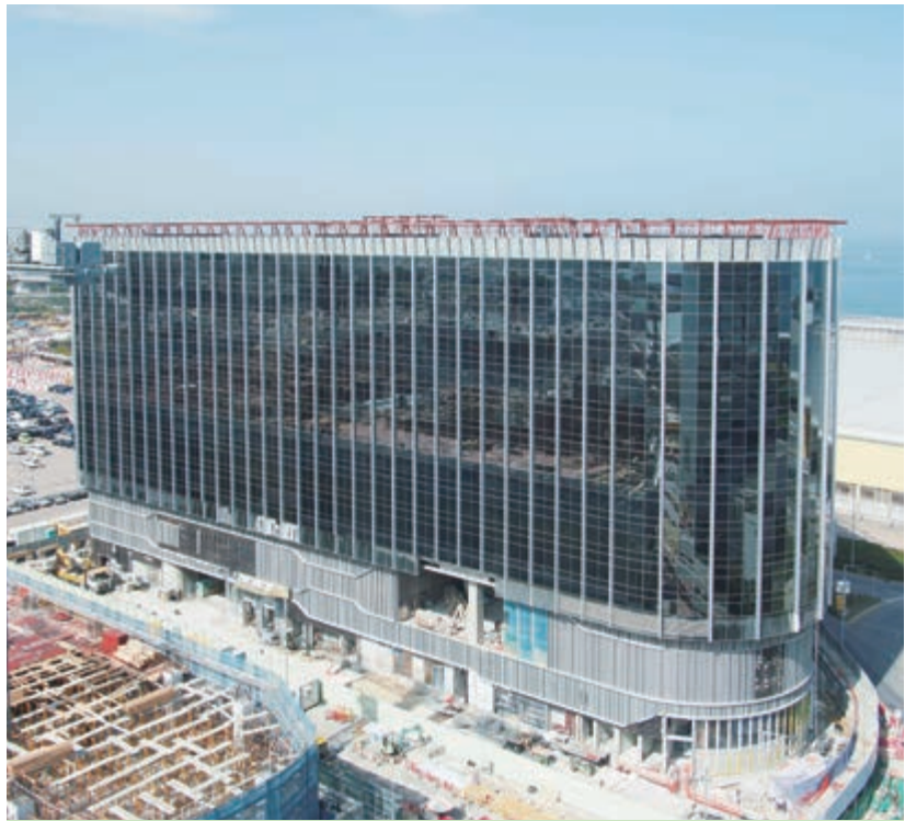
Regala Skycity Hotel - superstructure works completed
