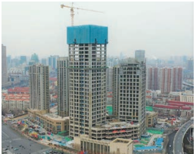
Office towers and commercial podium - superstructure works in progress
