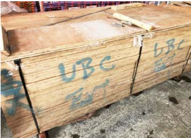
Timber collected at the construction site for recycling
