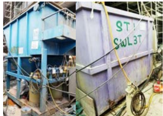
Wastewater treatment facilities at construction sites
