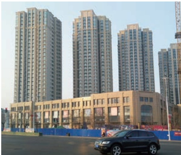
Residential towers and commercial complex of Regal Renaissance - completed
