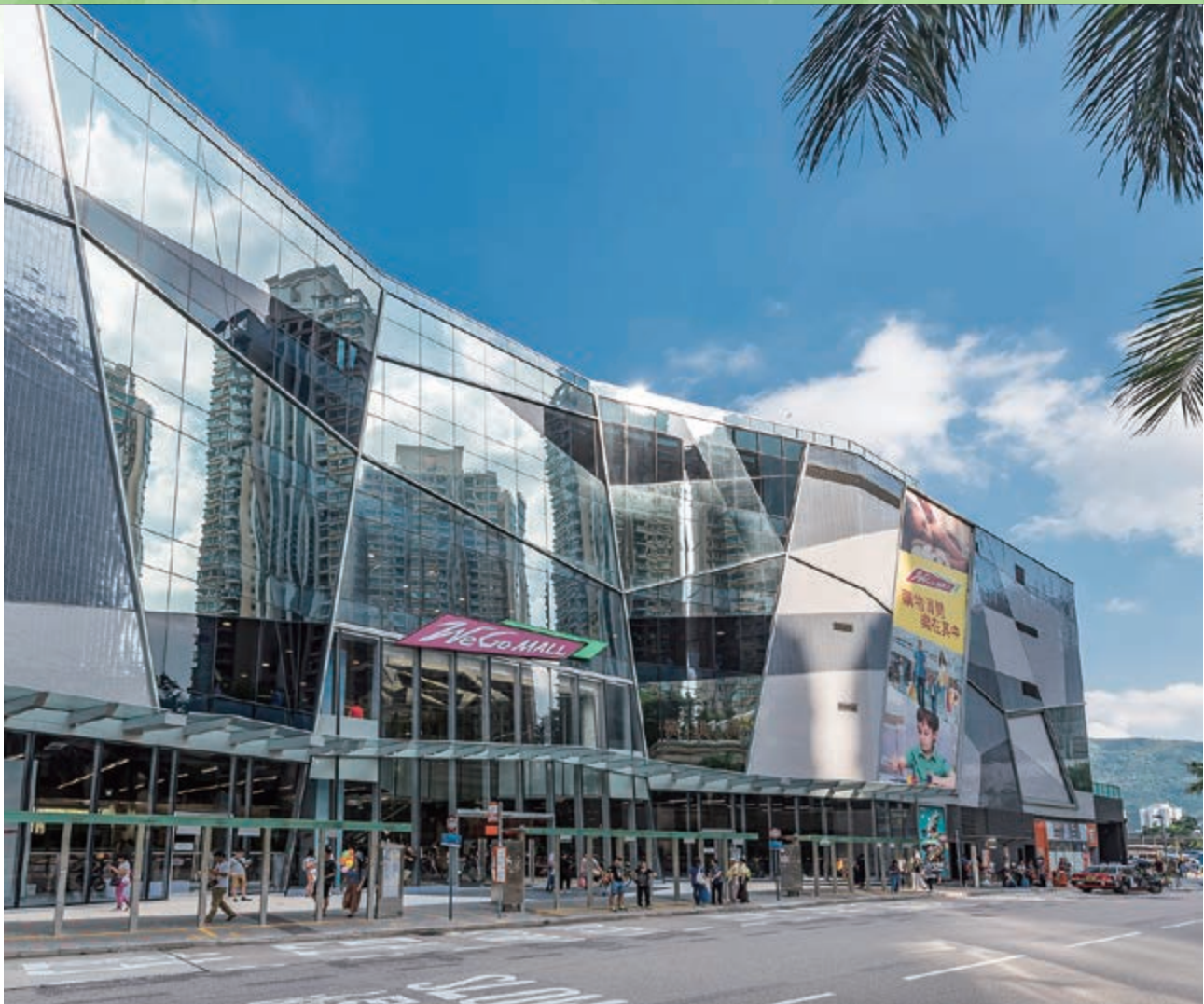
We Go MALL, a shopping mall at No. 16 Po Tai Street, Ma On Shan, Sha Tin, New Territories
