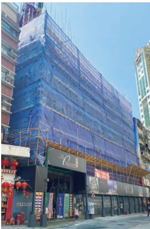
The Queens - superstructure works in progress
