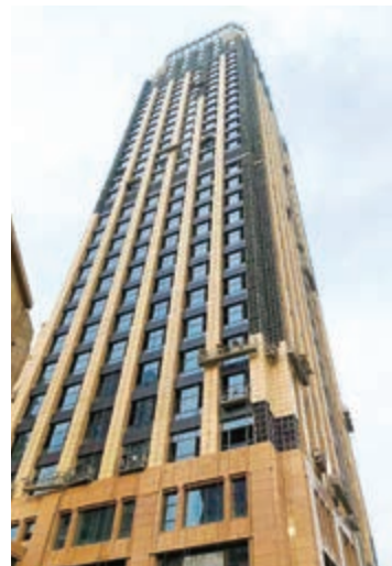
An office tower - superstructure works in progress
